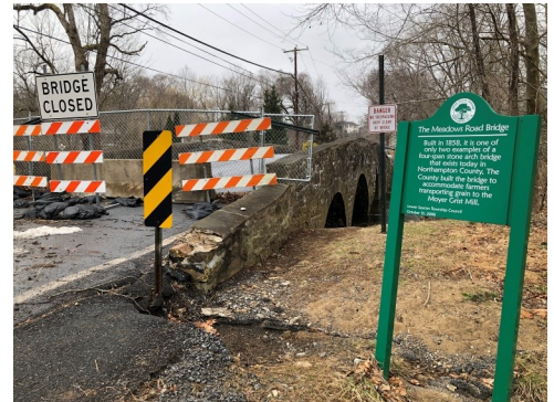
Meadows Road Bridge
