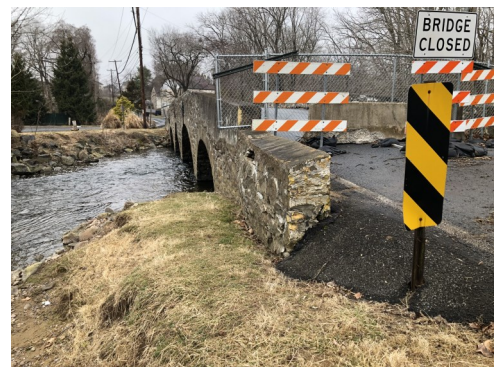
Meadows Road Bridge
