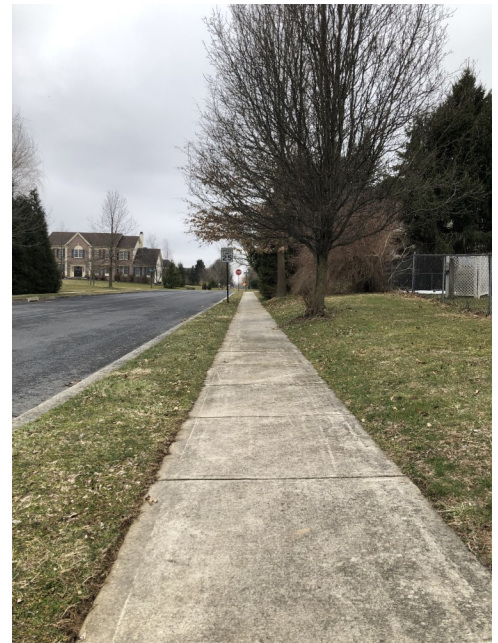
Existing sidewalk in a residential neighborhood
