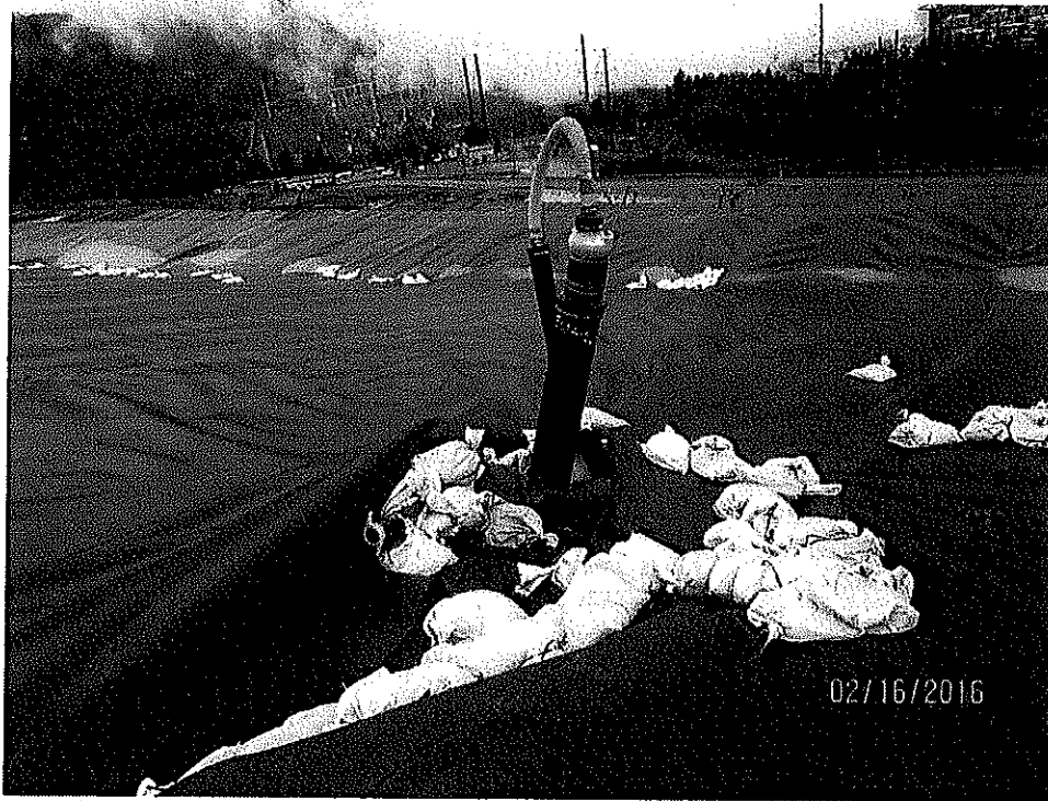
3. View of one (1) of the affected wells, showing that vacuum line has been reattached, liner has been cut, and sandbags have been placed.
