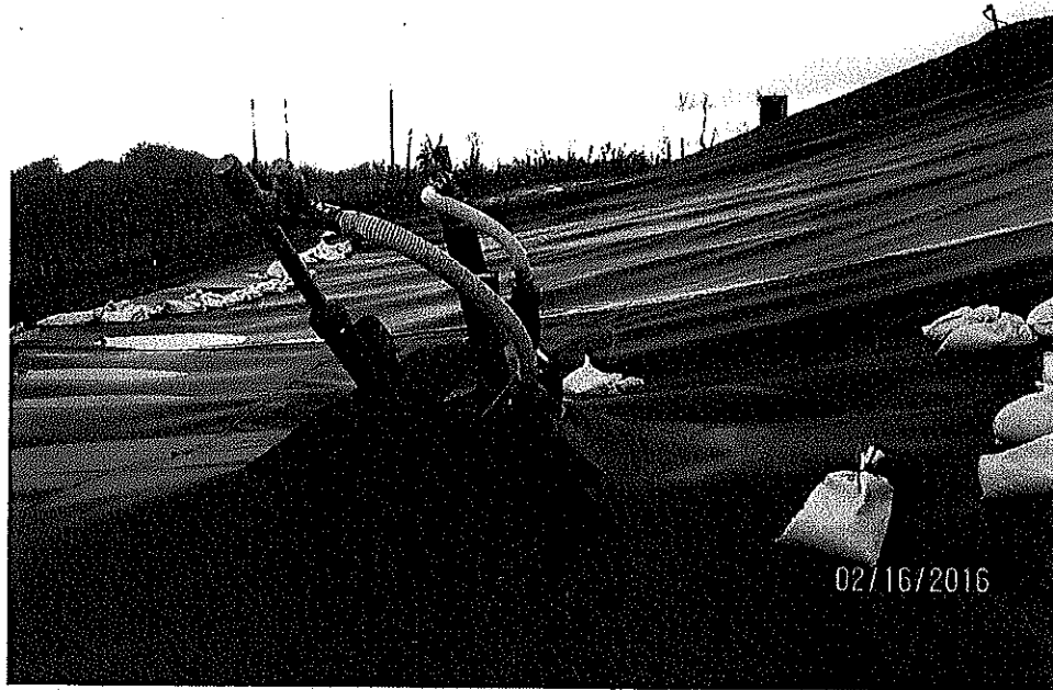
4. View of other two (2) affected wells, showing that vacuum lines have been reattached, liner has been cut, and sand bags have been placed. View is looking west (note LSA water tank in background).
