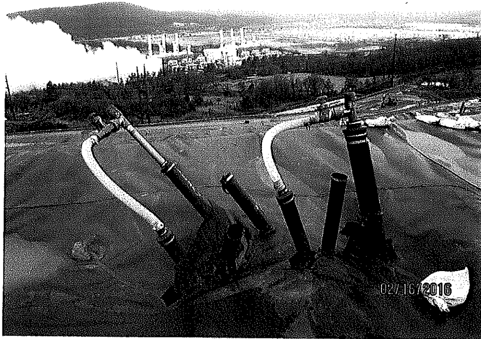
5. Additional view of affected wells.
